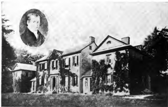
WELLS-STOKELY MANSION (Built in 1798 by Bezael Wells)
